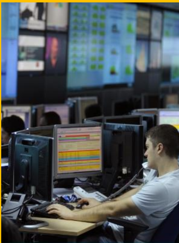
Network Operation Center
