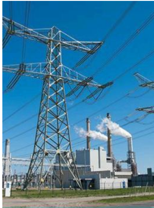
Utilities Process Control Centers
